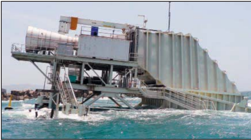
Concepts NREC installed its first wave energy platform off the coast of Australia. The turbine captures air pushed up into it as the waves move underneath and uses the oscillating air column to drive the turbine.
