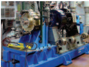
This custom gas-turbine test rig is installed in the client's facility.
