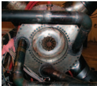
Standard rigs. Individual elements or complete stages can be tested in existing, standard rigs.
