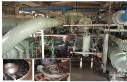
Figure: Rerated multistage, gear-driven centrifugal compressor. Various new impellers, diffusers, volutes and seals were introduced to meet new operating specifications
